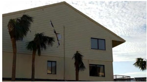
Wood plank siding (note wind-borne debris damage)
