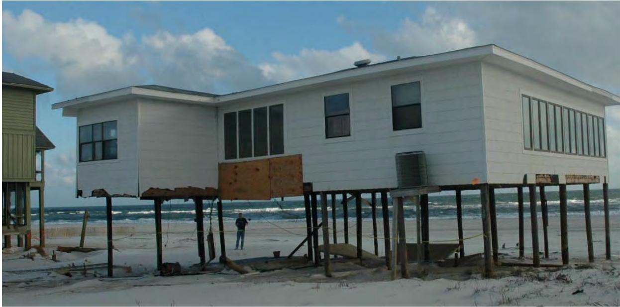
**Figure 29:** Missing or collapsed piles. (Photo Credit: US Army Corp of Engineers)
