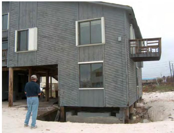
**Figure 28:** Scour around a foundation of a coastal single-family home.
