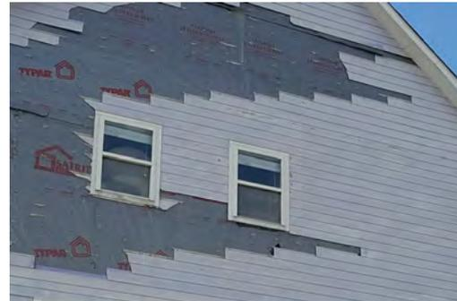
Fiber-cement board (note the failures along single planks)
