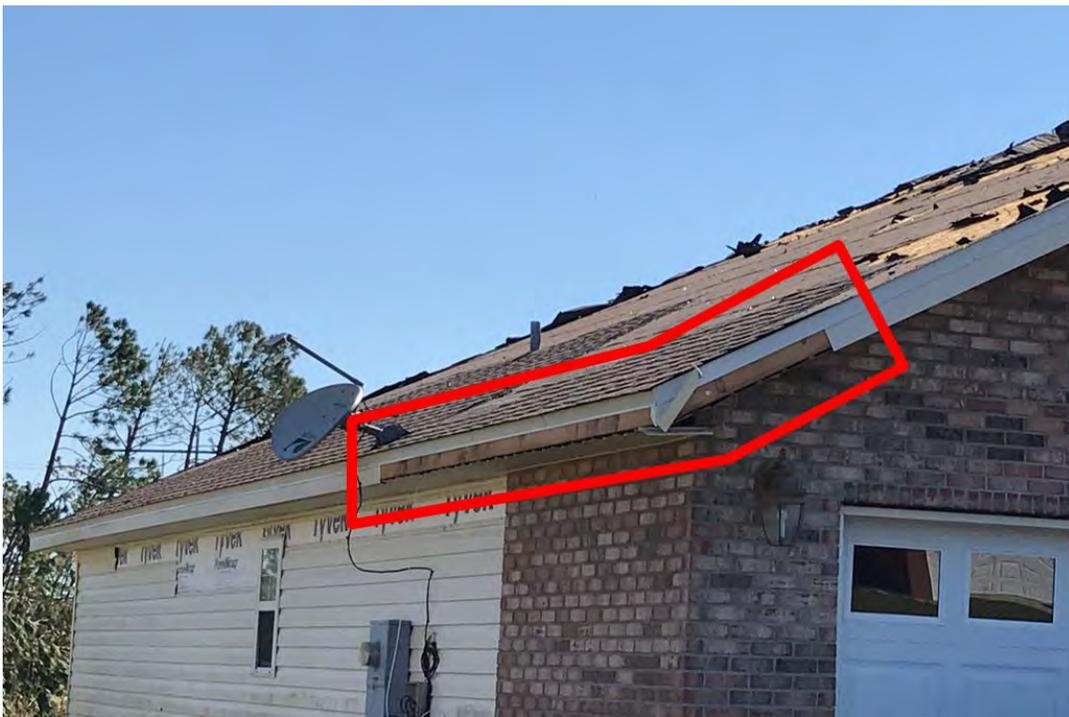
Figure 27: Example of fascia damage
