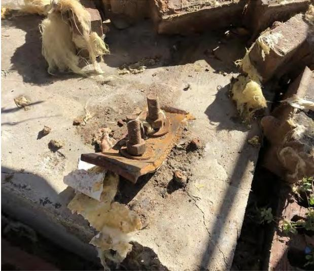
Anchor bolt with nuts and washers anchoring a failed column baseplate.
