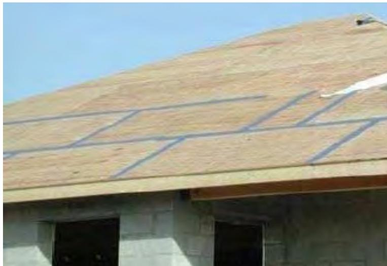
**Figure 25:** Peel and stick membrane over joints in the roof sheathing. (Photo Credit: [IBHS](#))
