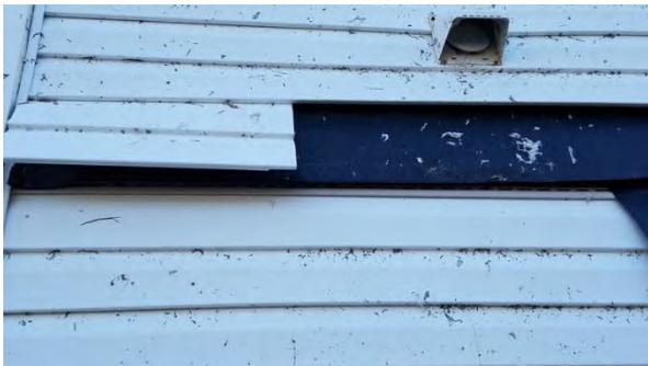
Vinyl Siding (note failures along double planks)
