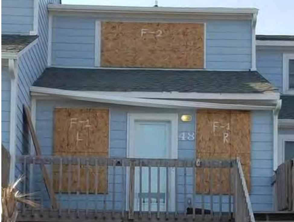
**Figure 26:** Labeled panels covering openings, indicating these were installed pre-storm.
