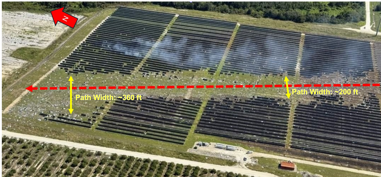
Figure 5.2. Tornado damage to the Lake Placid Solar Power Plant in Highlands County, FL (GPS: 27.333993, -81.360365). The tornado path and direction are indicated by the red dashed arrow. The tornado damage width was between 200-360 ft as it passed through the solar farm (Source: Duke Energy ).
