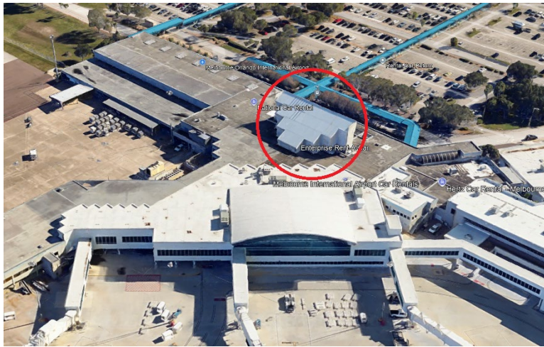
Figure 4.7. Aerial exterior view of the Melbourne Orlando International Terminal. The skylight that failed due to wind is circled in red (Source: Google Earth).
