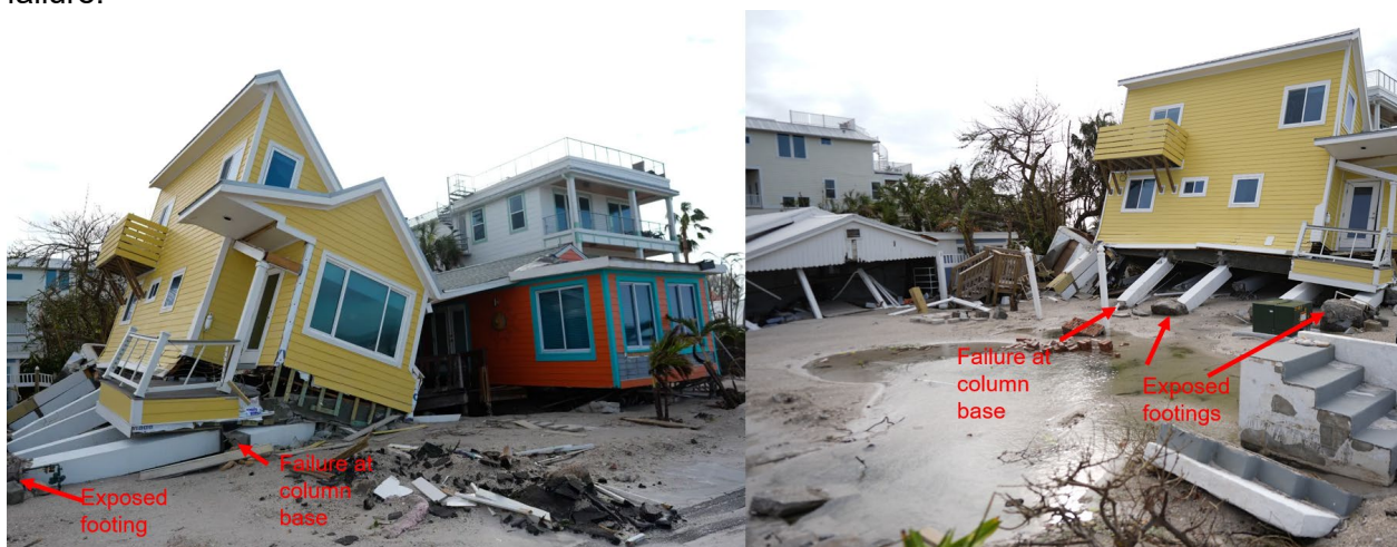
Figure 4.9. Overturned yellow elevated house on concrete piles on the barrier island of Bradenton Beach near Tampa Bay (Source: Rebecca Blackwell/AP ).
